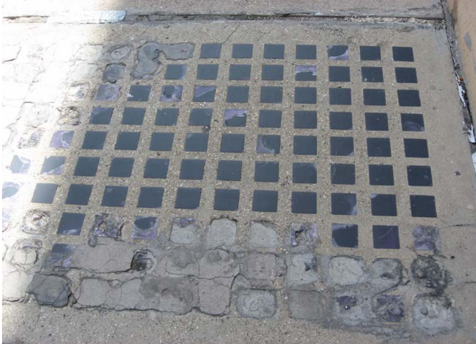
View of an individual panel. In the 1960's people began chipping and taking the glass thinking it was amethyst.
