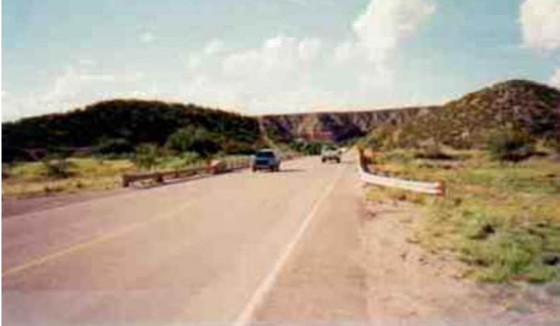
Figure 3. North bound Cotton Creek Bridge
