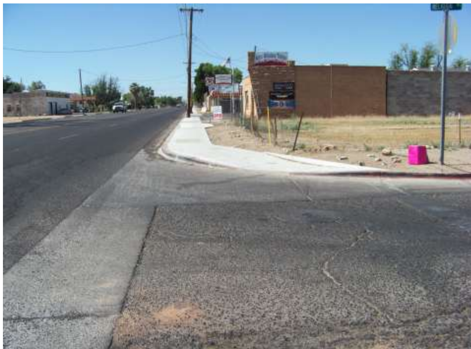
Photo #2: At Beginning of the Project: Relation Street (MP 120.33) looking south at newly completed sidewalk (Phase 1 – ARRA Project).
